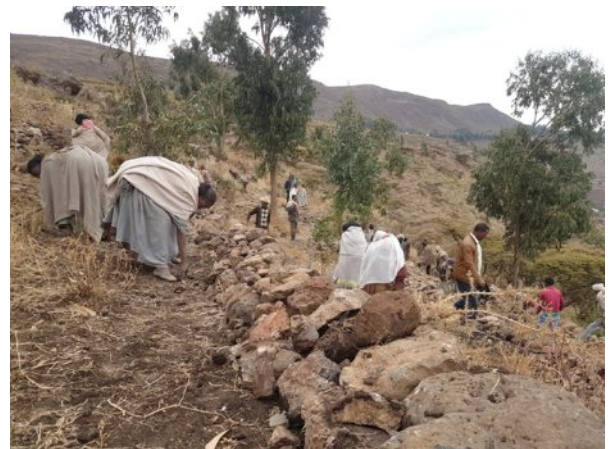
Figure 3. Constructing soil and water conservation structures
