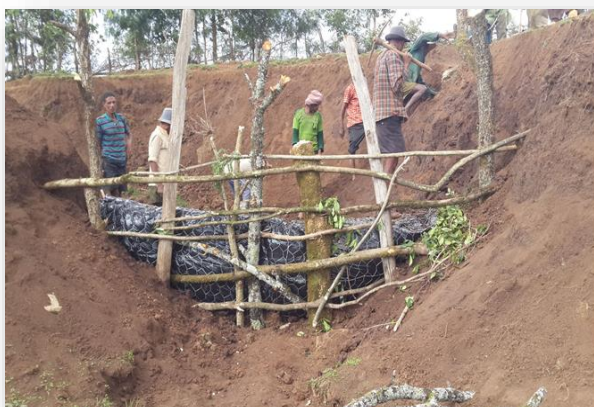
The two pictures illustrate the 'before' and 'after' scenarios of erosion management. On the left the construction and on the right the fully grown over vegetation slows water and reduces soil erosion. Note that they are not taken from the same site.
