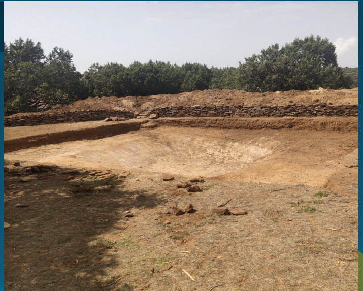
A water harvesting pond under construction.
